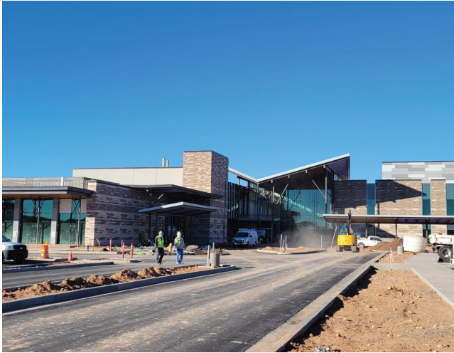
Pictured: Front entry construction of the Dilkon Alternative Rural Health Center in Dilkon, AZ. The center, serving the Navajo Nation, consists of over 30 departments and 600 rooms and offers emergency and diagnostic services. The facility was completed in February 2022.
